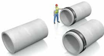
Position plain ended pipes.
